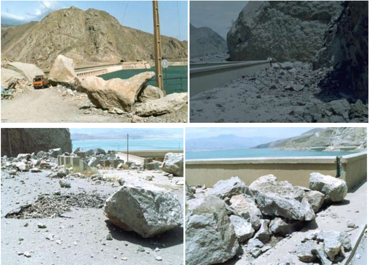
Fig. 11 : Rockfall at the dam site: Large displaced rocks above the spillway intake on left bank (top left)
