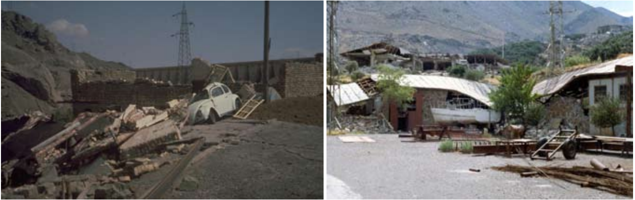
Fig. 13 : Collapsed buildings at dam site caused by strong ground shaking
