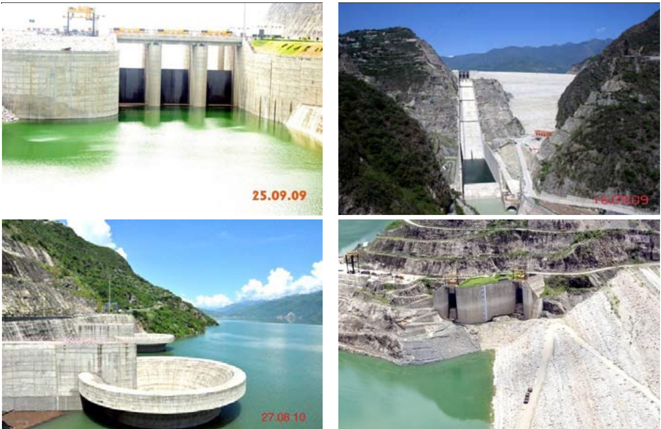
Fig. 3 : Chute (U/s & D/s), Right Bank & Left Bank Shaft Spillways (clockwise from top)
