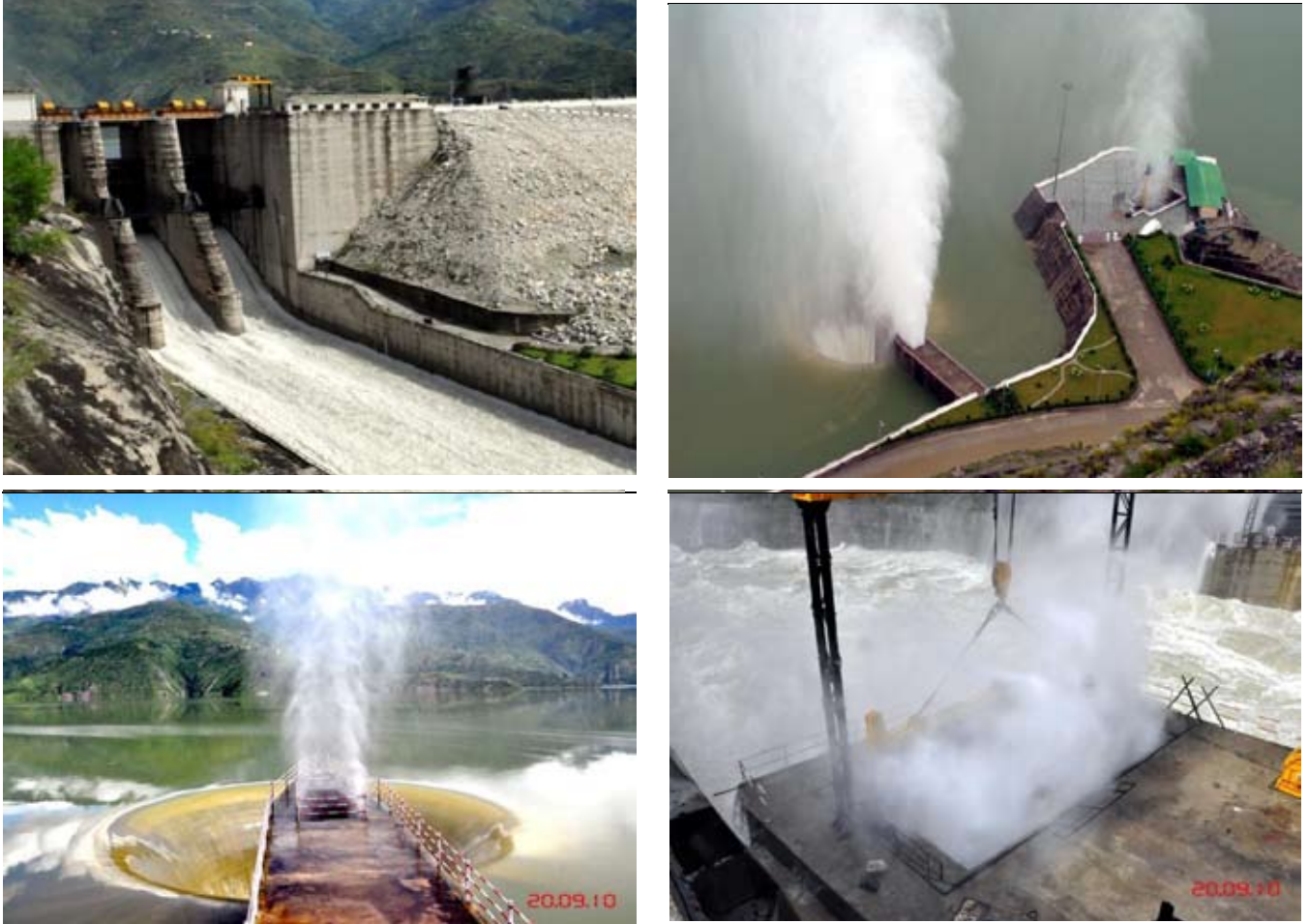
Fig. 4 : Spillways in Operation during 2010 Flood
